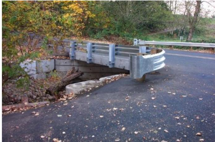
Several areas in the Township have missing, damaged, or aged guiderail that needs to be addressed. Most locations planned for guiderail are areas where the shoulder of the road drops off sharply. Guiderail repairs are replaced intermittently in critical areas when damaged. However, replacing aged guiderail and adding guiderail to new locations is expected to create an economy of scale when bidding the work to contractors. Operating costs are not expected to be impacted significantly.
