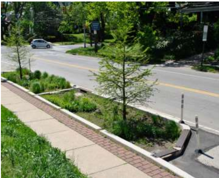
Image 17. Example of a stormwater bump out in East Falls Philadelphia which serves to mitigate flooding on the roadway and calm traffic.
