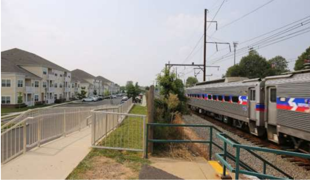
Image 7. The Station at Bucks County, located in Warminster, Pennsylvania is a prominent example of providing residences near transit options, a strong possibility for Langhorne Station. The 16-acre property includes 233 one- and two-bedroom rental units.
