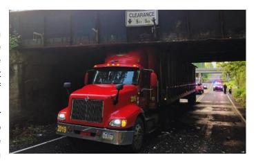
A mast arm is proposed to be repurposed to this area to provide large vehicle operators with more advanced notice. A study to identify a solution in this area is proposed in future years. This study would recommend the best method to prevent trucks from getting stuck.
